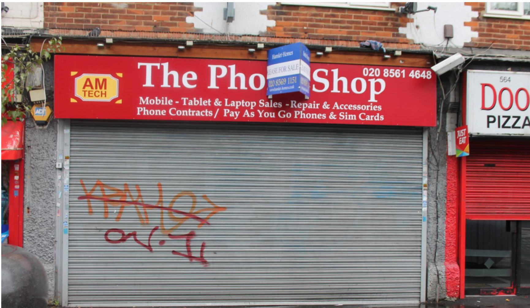
The Phone Shop, Uxbridge Road, Hayes, UB4
